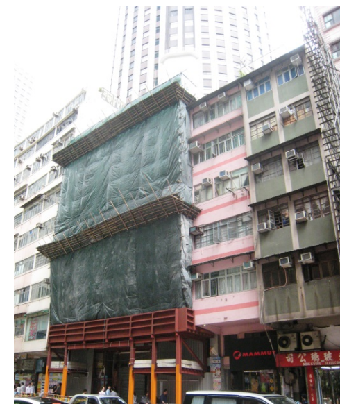
155-159 Queen's Road East – Demolition works
