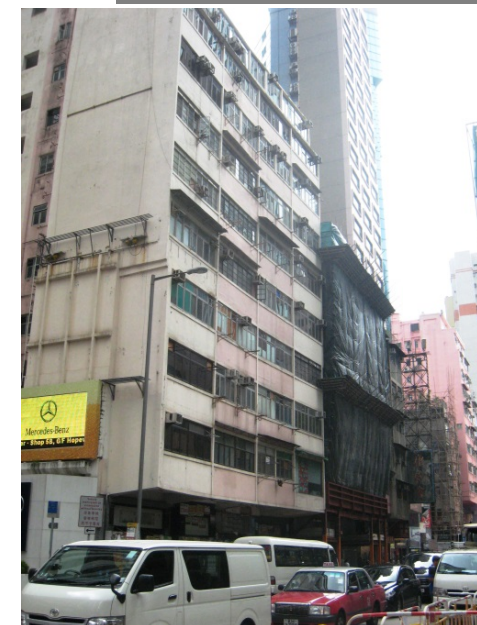
161-167 Queen's Road East
