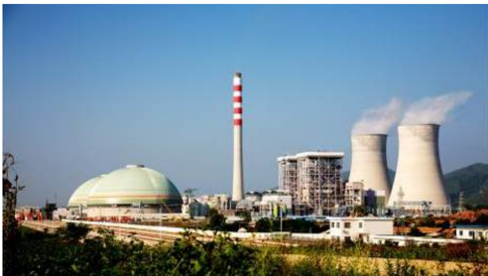
Heyuan Power Plant
